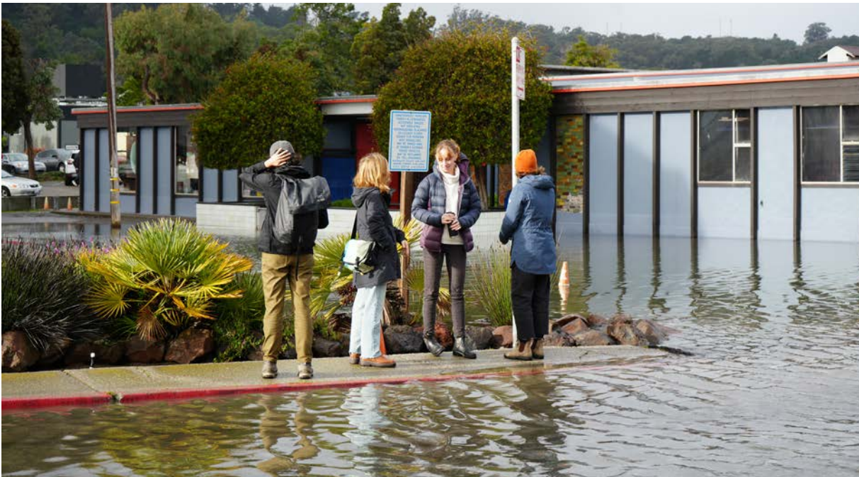
Gate 5 Road already experiences significant flooding during king tides as shown here. In the future, concerns related to flooding and continued land subsidence increase the need for adaptation.
