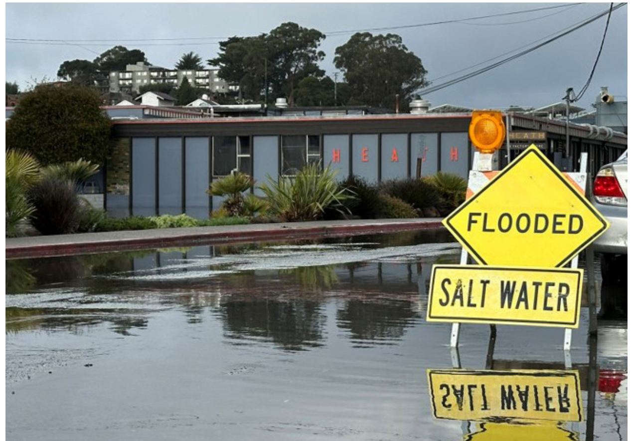
Flooding is already a challenge along Gate 5 Road.
