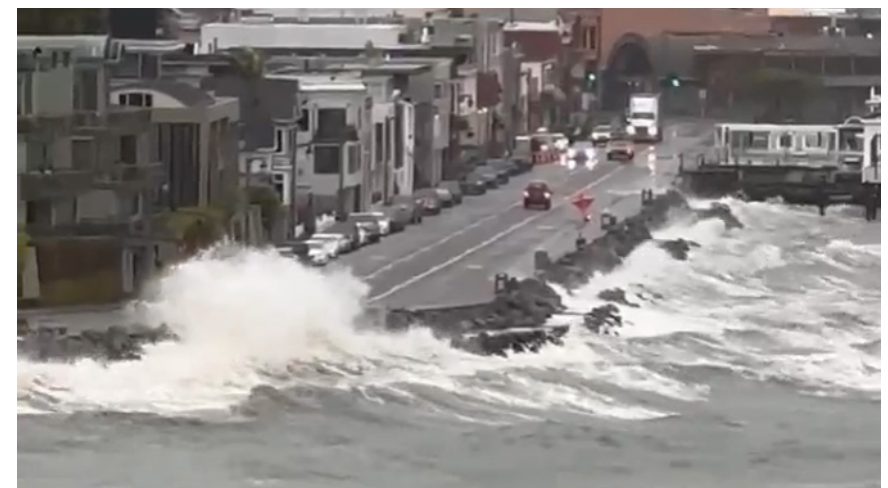
Wave over-topping along the promenade during storm
