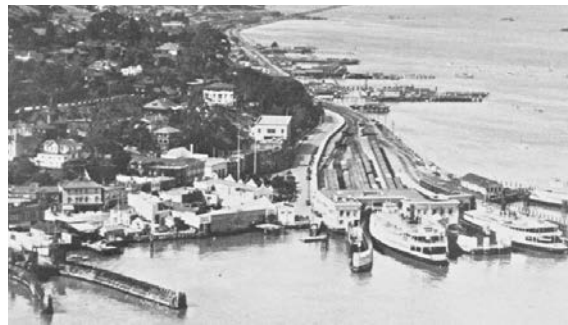
Historic photo of Sausalito's Ferry Terminal
